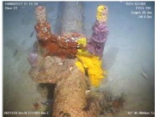
Image 2. Rock bolts secure the GEP in some sections to increase pipeline stability
