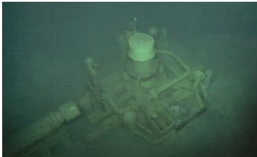
Typical well flowbase
