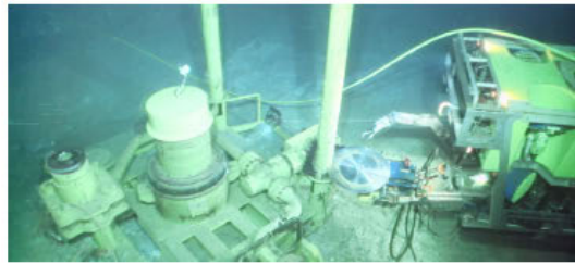
Typical subsea cutting activity
