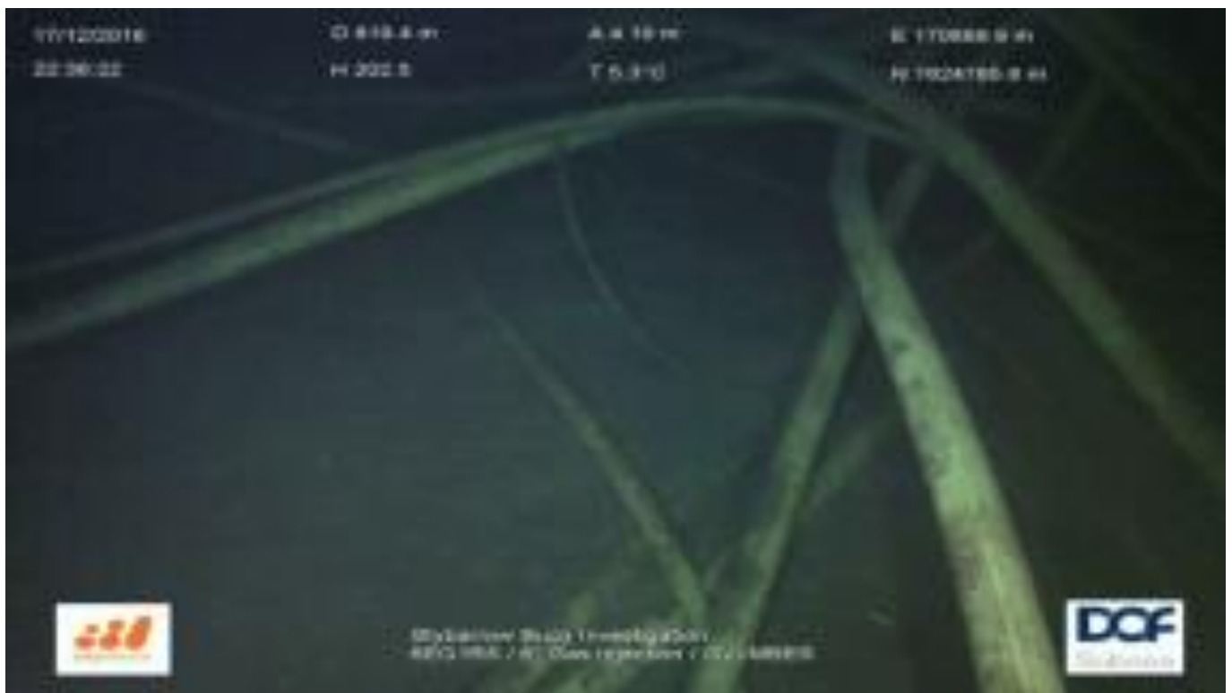
Figure 3-8: Tangled risers on seabed near the DTM buoy
