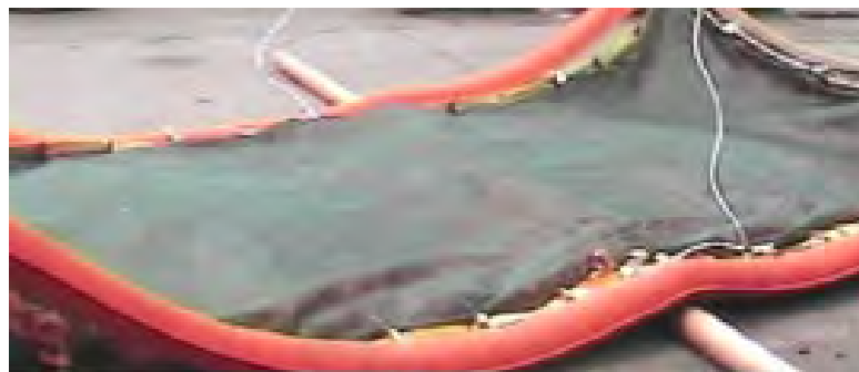
Figure 2-20: Example of weighted edge soft mattresses (with fronds)
