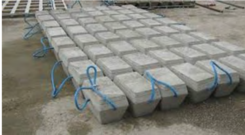
Figure 2-19: Example of concrete mattress
