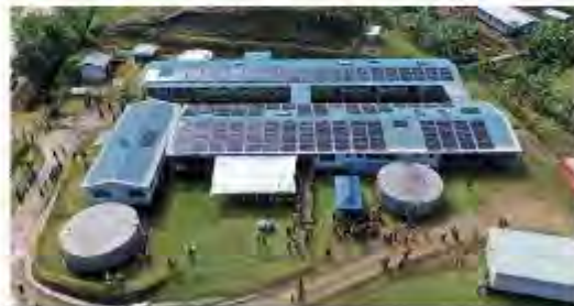
Worked with US AID to deliver solar power to Pimaga Hospital
