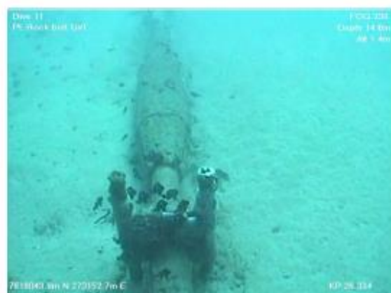
Image 3. Partially buried section of the GEP with rock bolts
