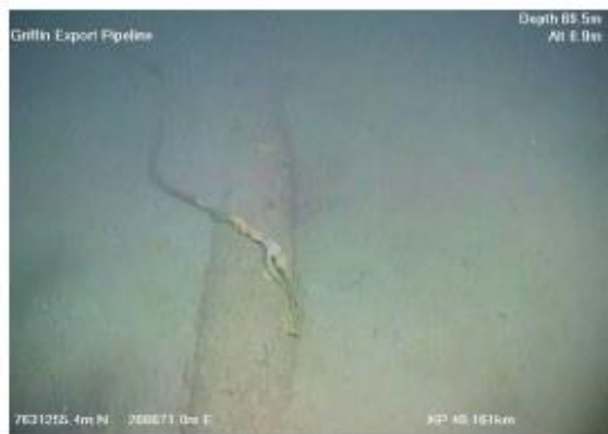
Image 1. Partially buried section of the GEP
