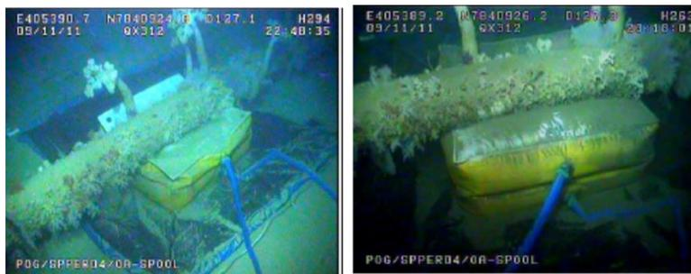
**Figure 3-9: Grout bags in position**
