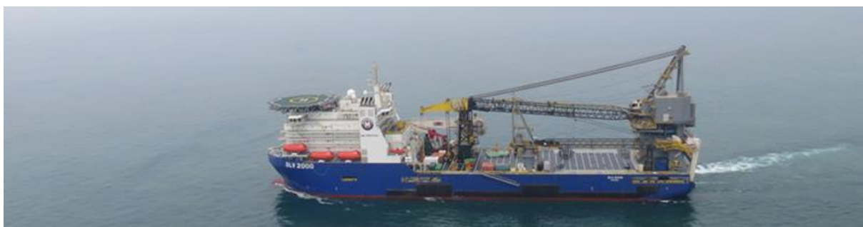
Figure 4. DLV 2000 – the construction vessel considered (McDermott 2018).
