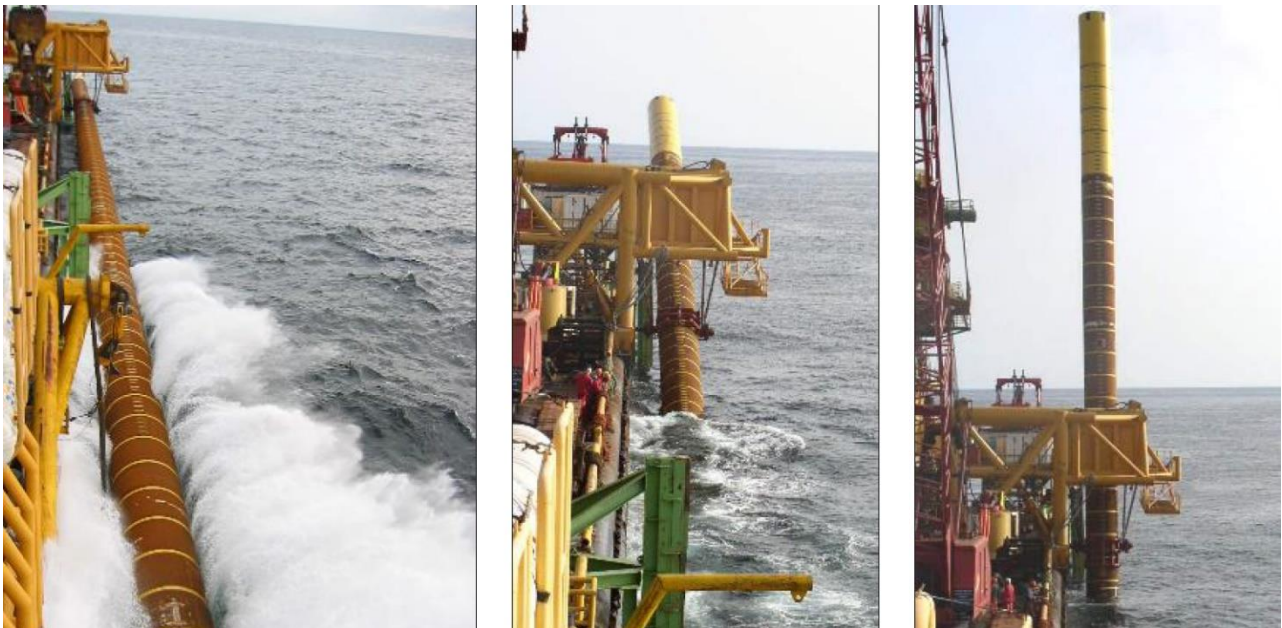
Figure 6-20: Example of Primary Pile Upending (Pin and Collar Method)
