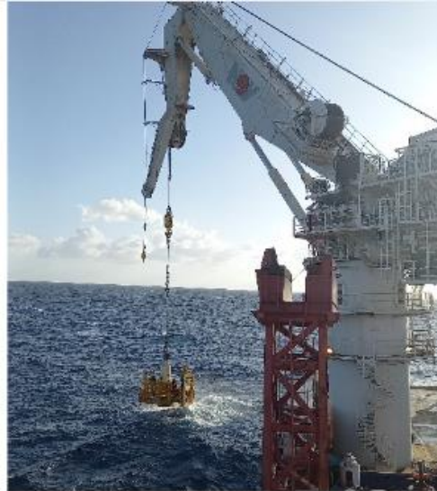
Figure 3. Typical Subsea Equipment Recovery Activity
