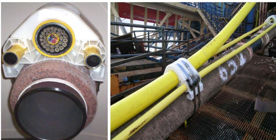
Figure 3-6: Minerva Pipeline Bundle
