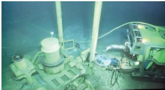
Figure 2. Typical Subsea Cutting Activity
