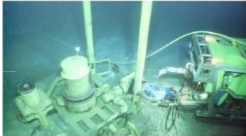
Figure 2. Typical Subsea Cutting Activity
