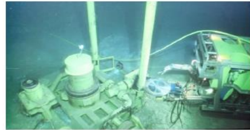
Figure 3. Typical Subsea Cutting Activity
