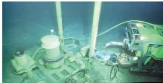
Figure 3. Typical Subsea Cutting Activity
