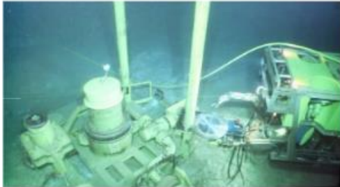
Figure 2. Typical Subsea Cutting Activity
