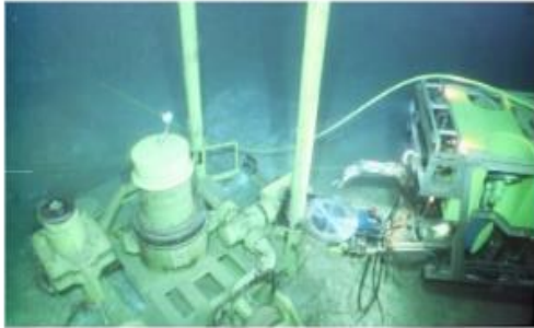
Figure 2. Typical Subsea Cutting Activity
