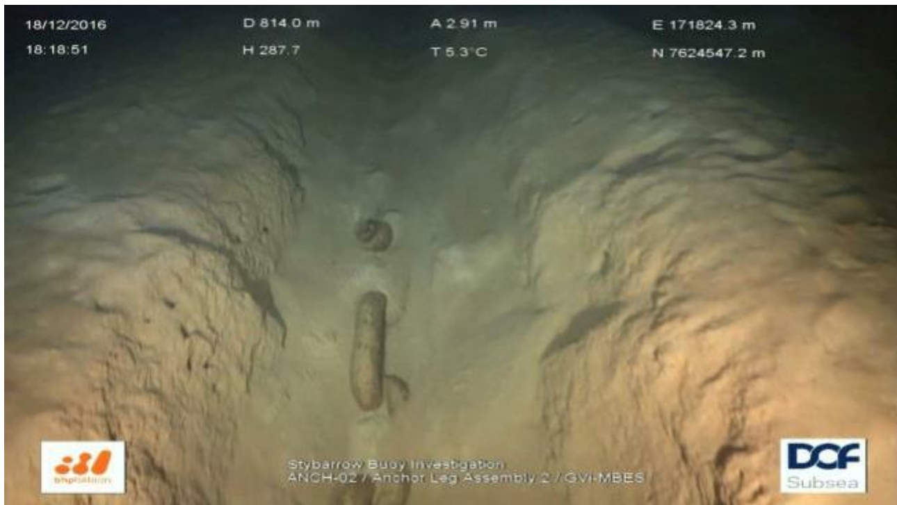
Figure 4-5: Partially buried chain at mooring leg touchdown point (bottom/heavy chain in Figure 4-4) showing degree of burial several hundred metres from the associated anchor
