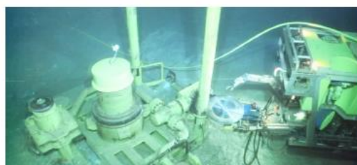
Typical subsea cutting activity
