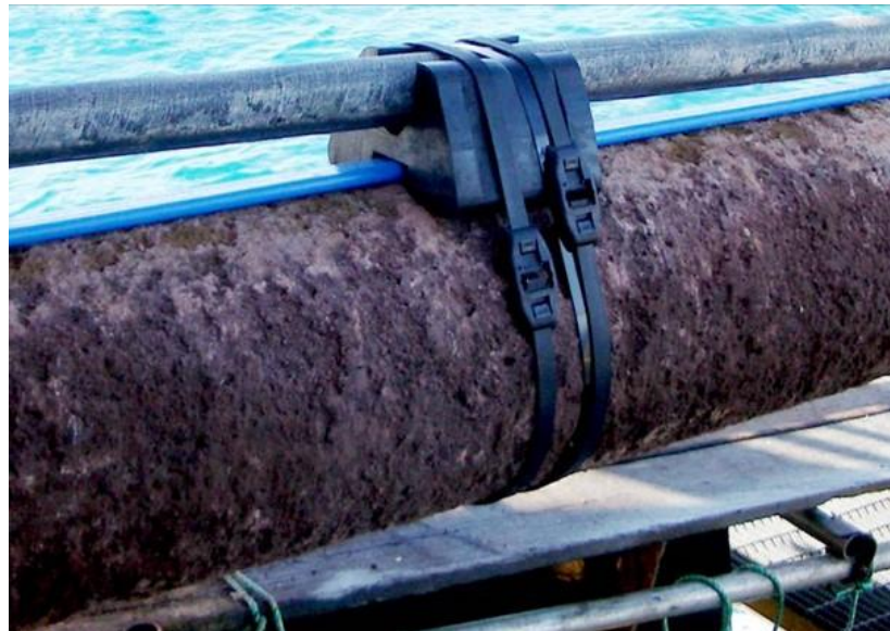
Figure 2.3: Chemical and power umbilical attached to Production Pipeline.
