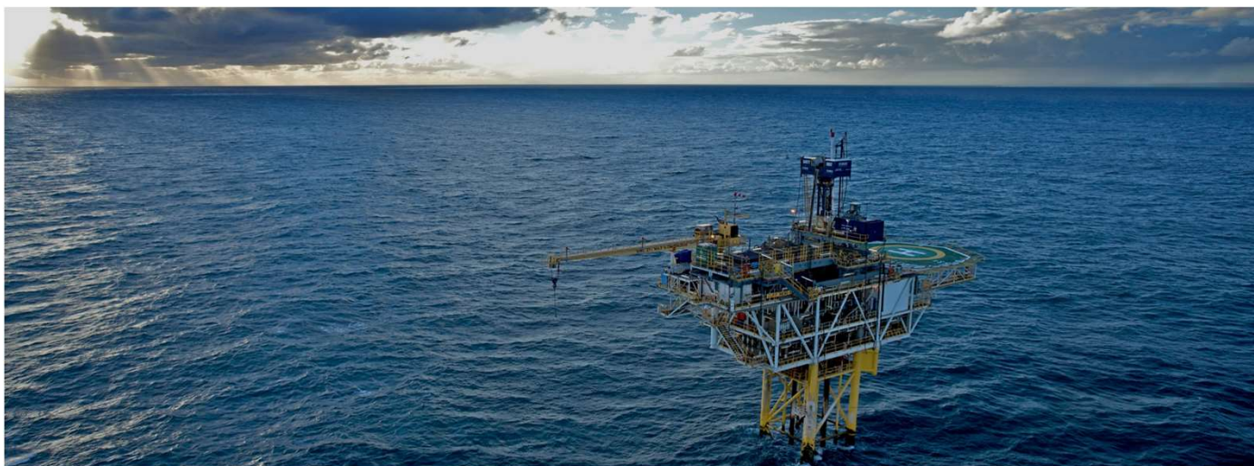
FIGURE 1. Cliff Head Alpha Offshore Platform
