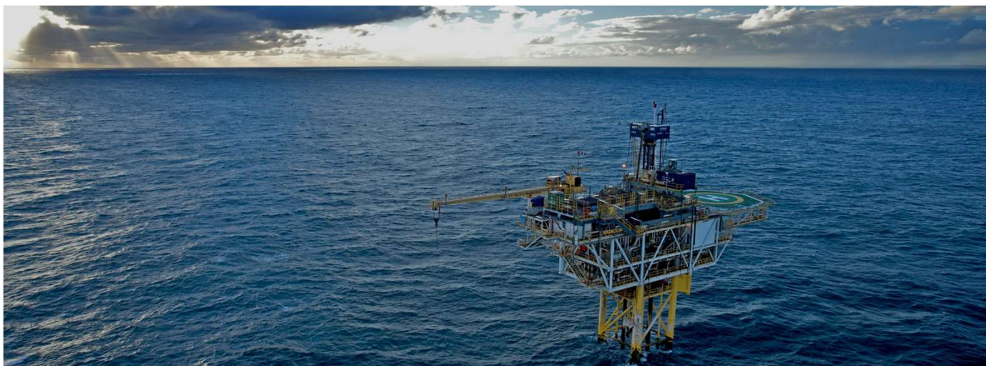
FIGURE 1. Cliff Head Alpha Offshore Platform
