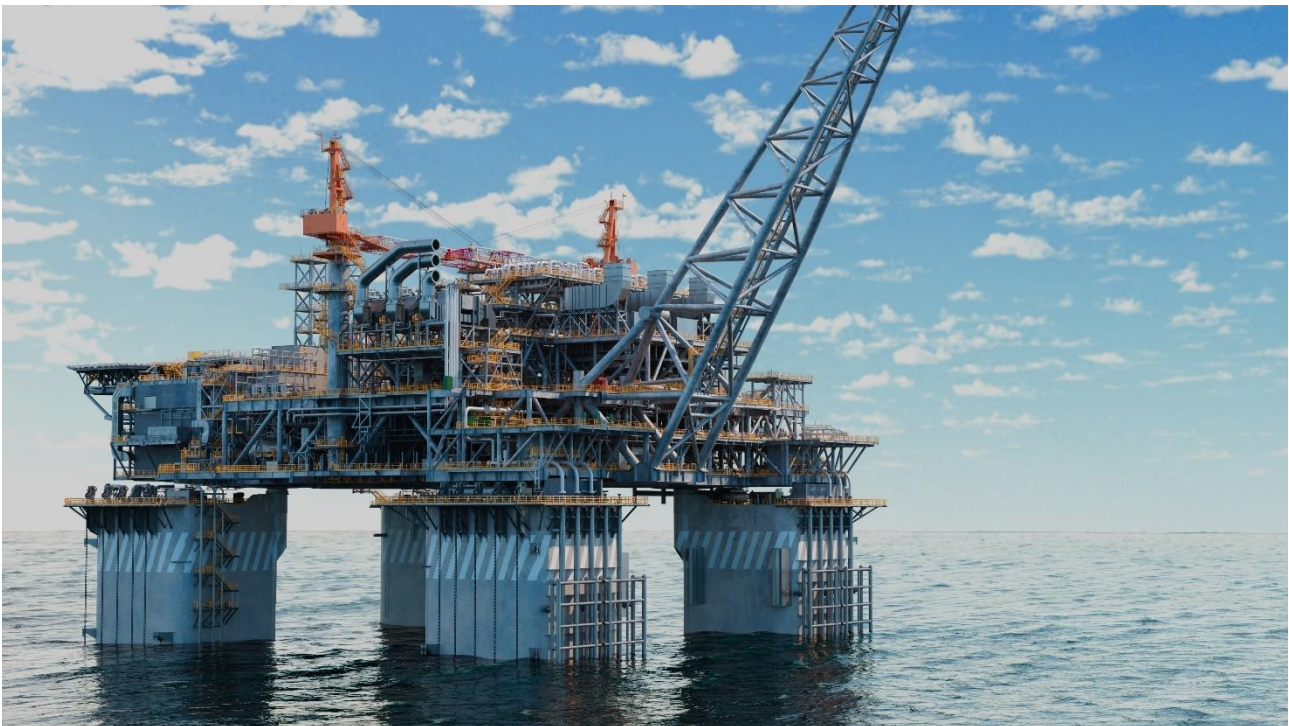
Figure 3-1: Scarborough floating production unit
