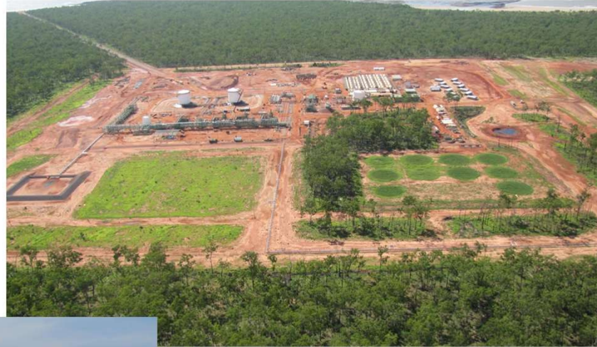
Yelcherr Gas Plant (YGP)
