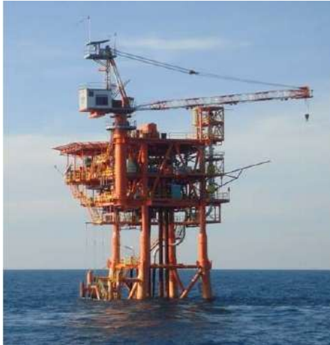
Wellhead Platform (WHP)
