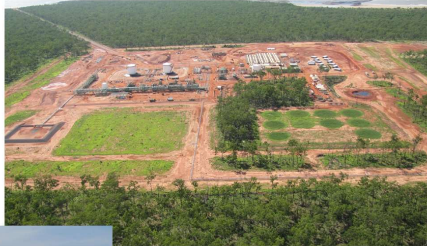
Yelcherr Gas Plant (YGP)
