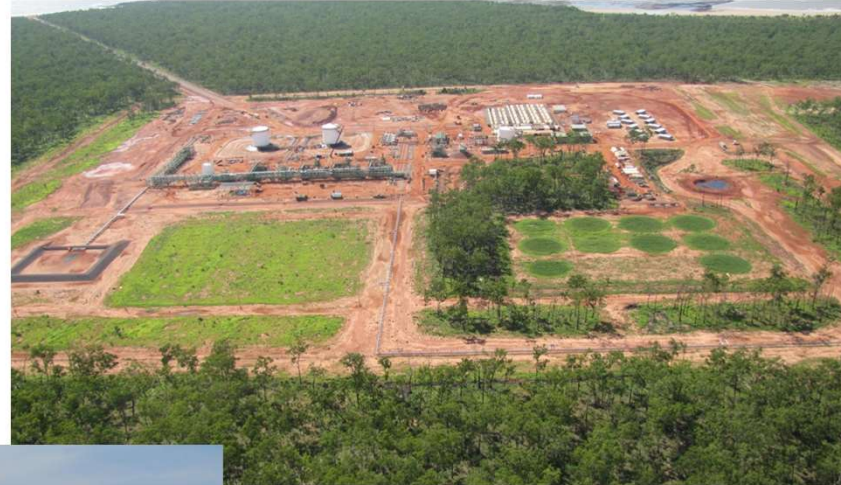
Yelcherr Gas Plant (YGP)
