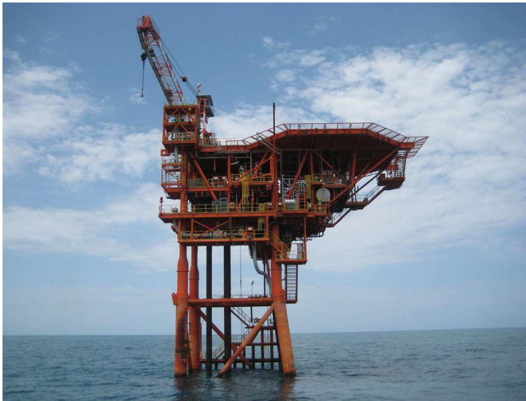
Figure 3.2: Blacktip wellhead platform
