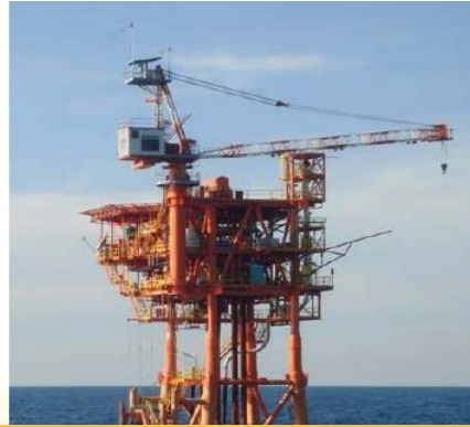
Wellhead Platform (WHP)
