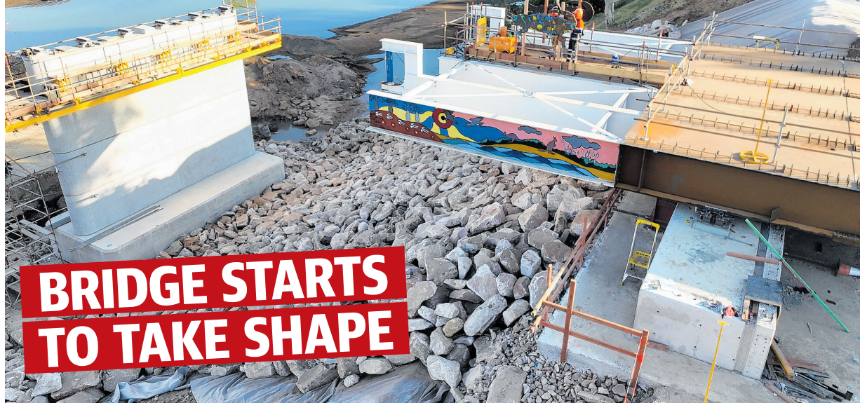
The first segment of the new bridge deck. Picture: Facebook
