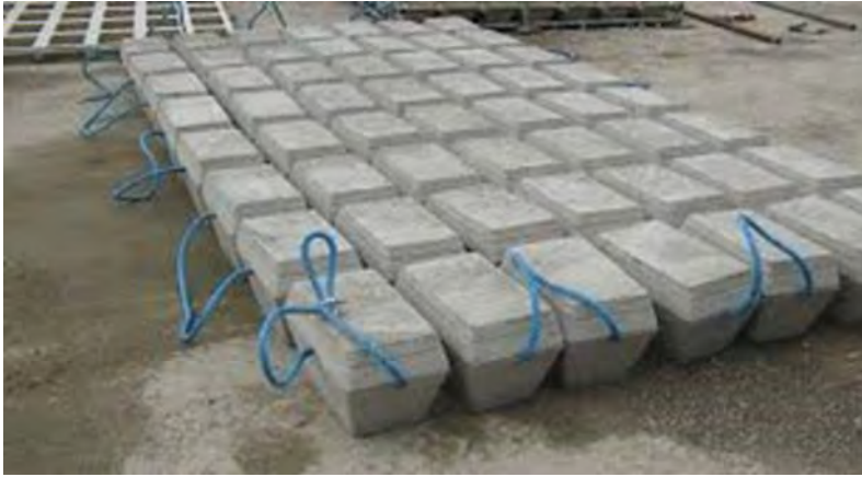
Figure 2-6: Example of a concrete mattress
