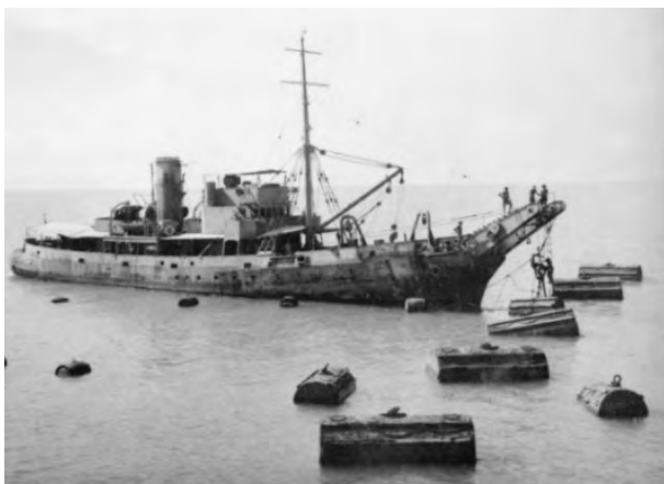
Figure 12: Boom vessel working on the Darwin anti-submarine boom net – showing detail of the net and buoys. 58
