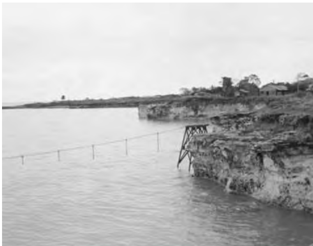
Figure 15: Anti-submarine boom net pylon, East Point. 65
