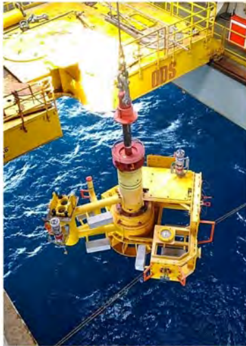
Installing the Wellhead
