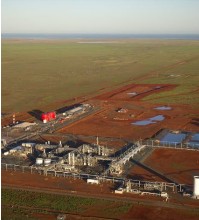
Devil Creek Gas Plant
