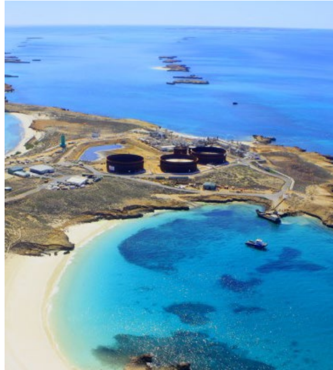
Varanus Island Gas Plant
