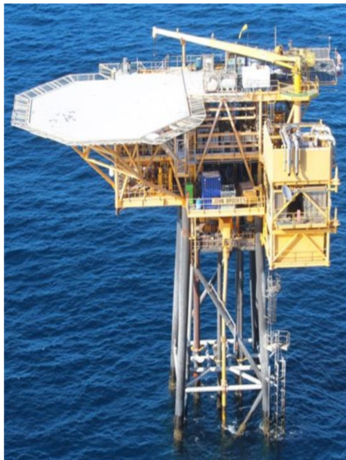
Figure 2.3: John Brookes wellhead platform – Halyard wing deck
