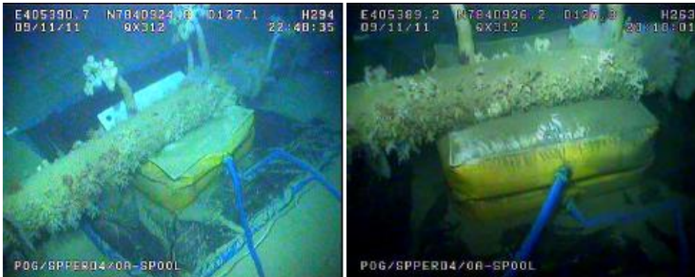
Figure 3-9: Grout bags in position
