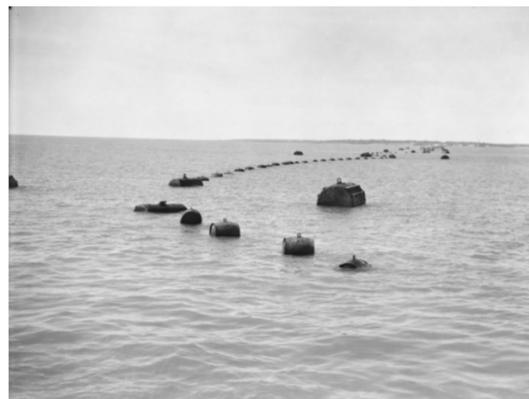
Figure 13: Darwin anti-submarine boom net – showing gates opening to allow the passage of a ship. 59
