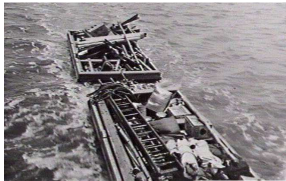
Figure 96: "Barges with materials for leper station being towed across harbour" 1937. 118
