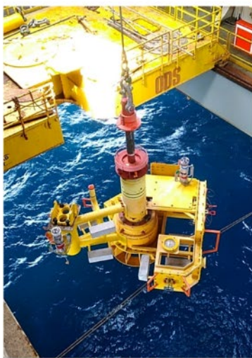
Installing the Wellhead
