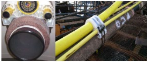
Figure 1. Minerva Pipeline Bundle Arrangement
