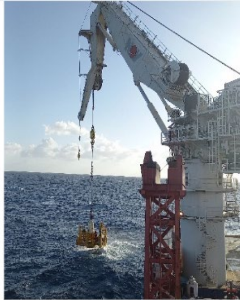
Figure 3. Typical Subsea Equipment Recovery Activity
