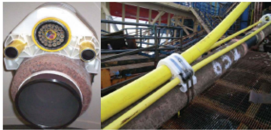
Figure 2. Minerva Pipeline Bundle Arrangement
