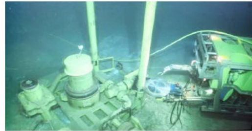
Figure 3. Typical Subsea Cutting Activity
