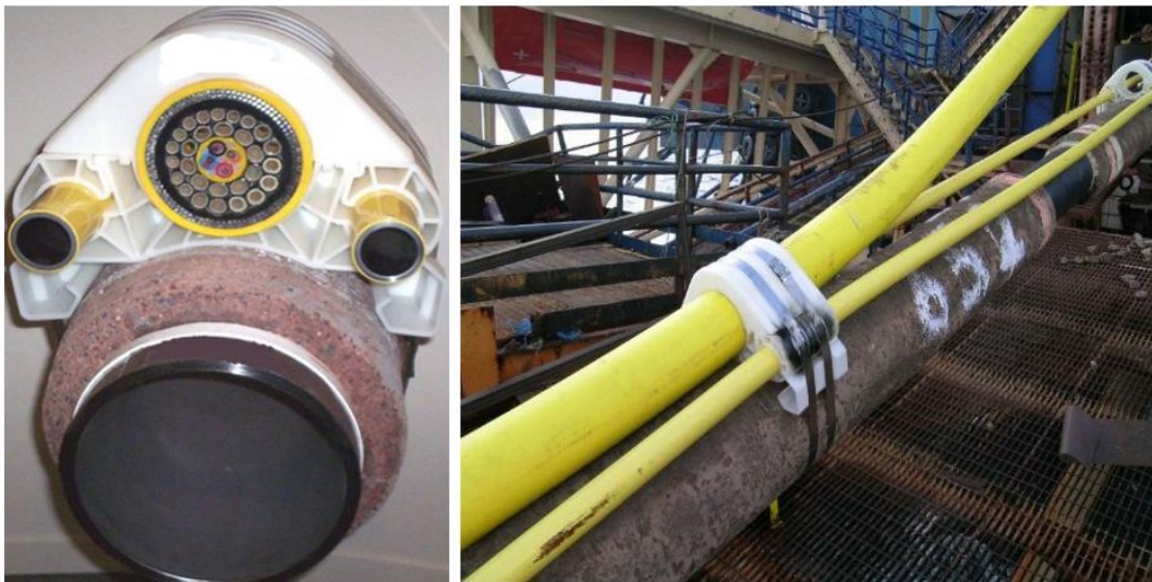
Figure 3-7: Minerva Pipeline Bundle
