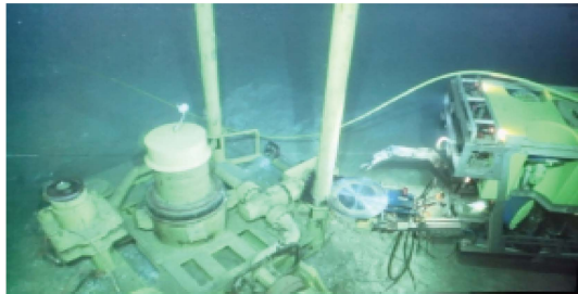
Figure 3. Typical Subsea Cutting Activity
