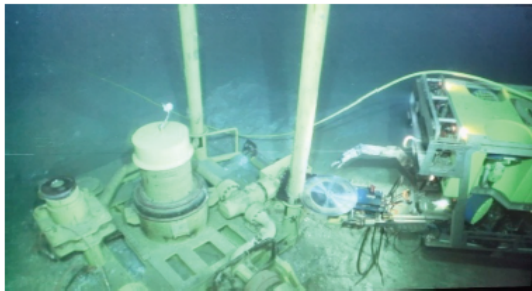
Figure 2. Typical Subsea Cutting Activity
