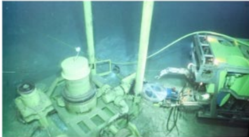
Figure 2. Typical Subsea Cutting Activity
