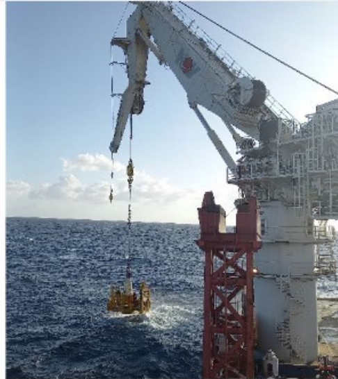
Figure 3. Typical Subsea Equipment Recovery Activity
