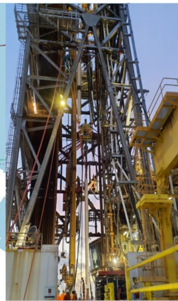
Derrick structure on drill rig
