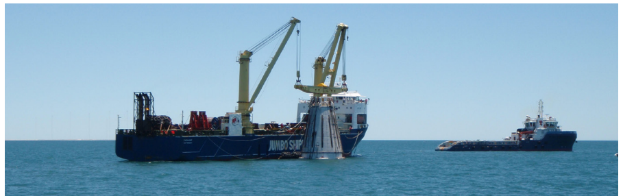
Image 1. Installation of the DTM in 2008
