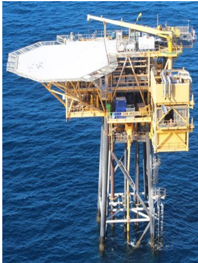
Figure 2-3: John Brookes wellhead platform – Halyard wing deck
