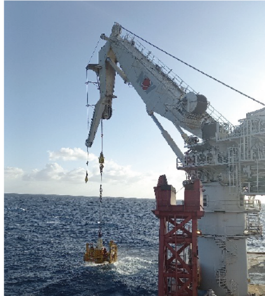
Figure 3. Typical Subsea Equipment Recovery Activity
