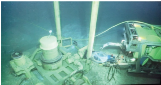
Figure 2. Typical Subsea Cutting Activity
