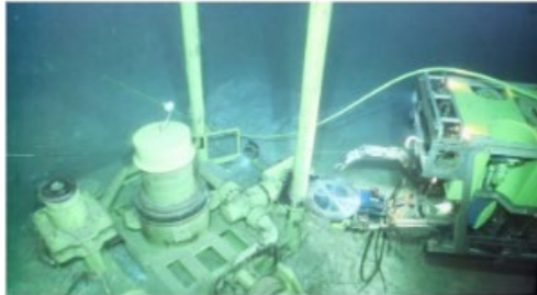
Figure 2. Typical Subsea Cutting Activity
