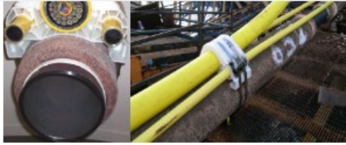
Figure 1. Minerva Pipeline Bundle Arrangement
