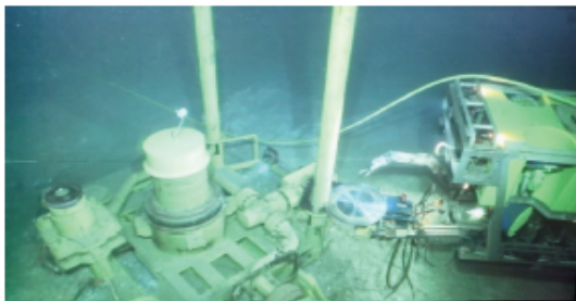
Figure 3. Typical Subsea Cutting Activity
