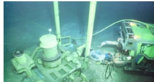
Figure 3. Typical Subsea Cutting Activity
