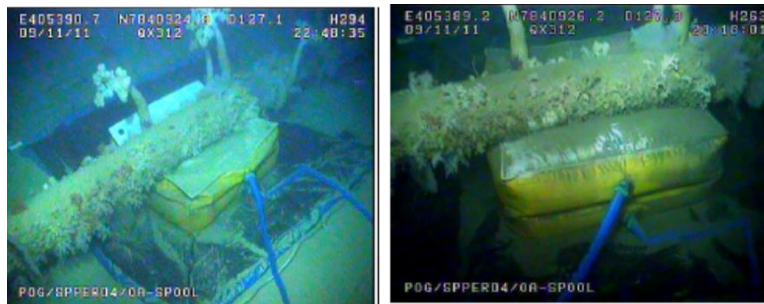
Figure 3-9: Grout bags in position
