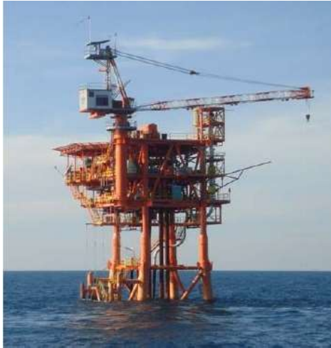
Wellhead Platform (WHP)
