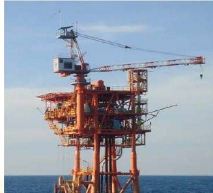
Wellhead Platform (WHP)
