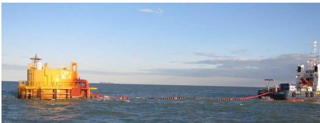
Figure 3.7: Single point mooring and floating hose
