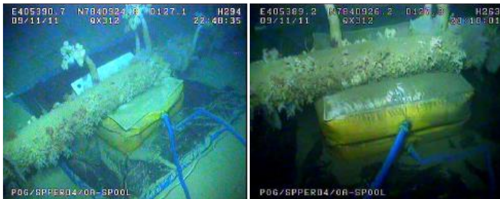
Figure 3-10: Grout bags in position
