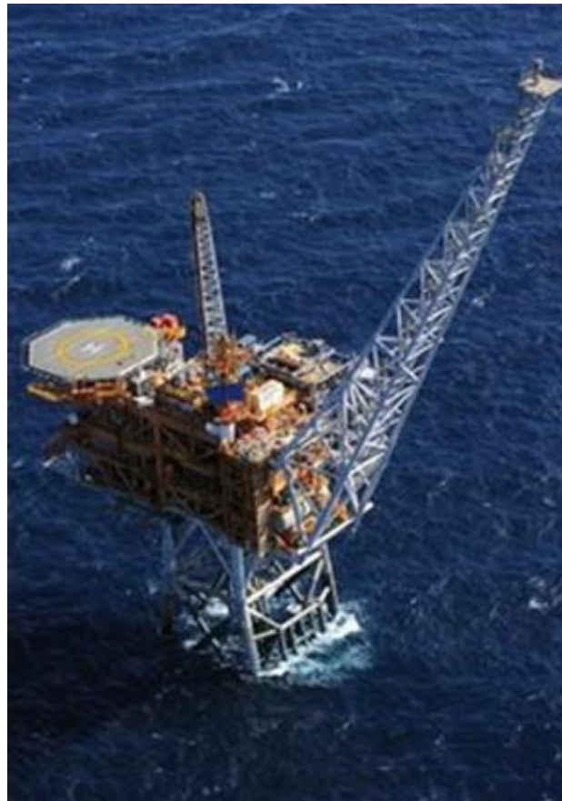
Figure 3-2: Photograph of the Pluto Alpha riser platform
