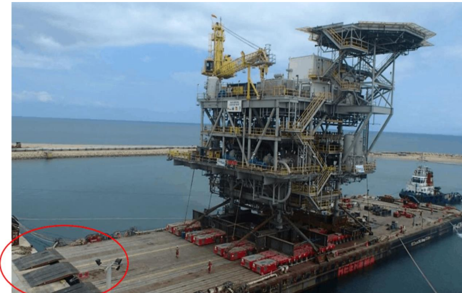
Topside load in using SPMTs with ramps
