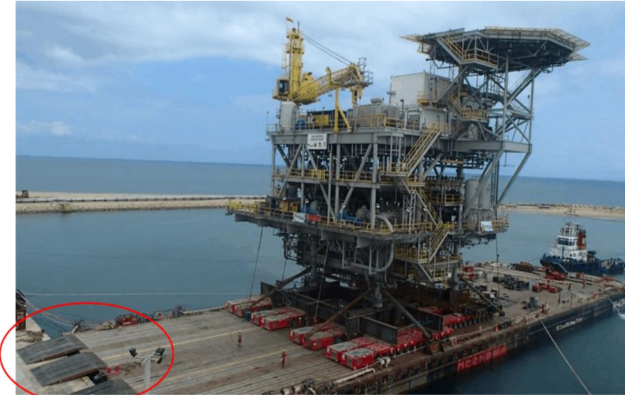
Topside load in using SPMTs with ramps
