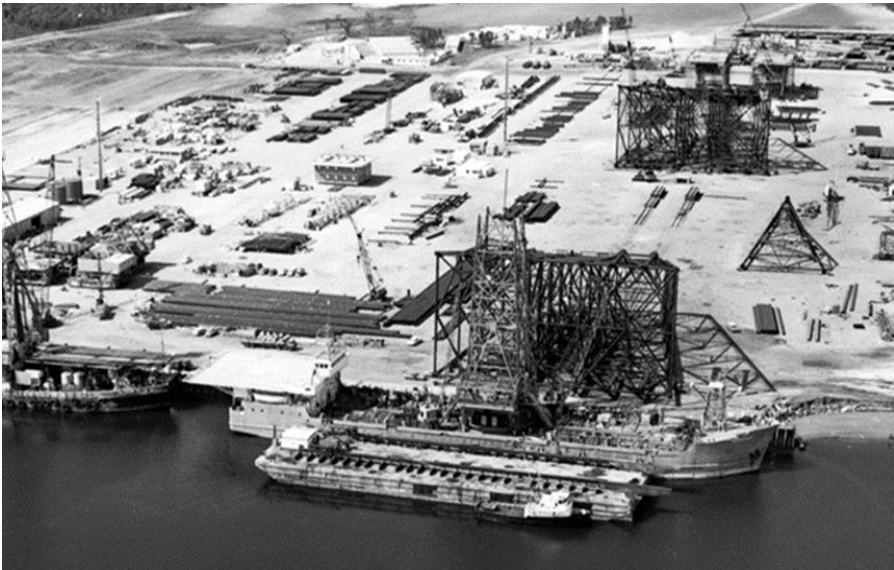
1970s jacket load out to Heavy Transport Vessel from BBMT
