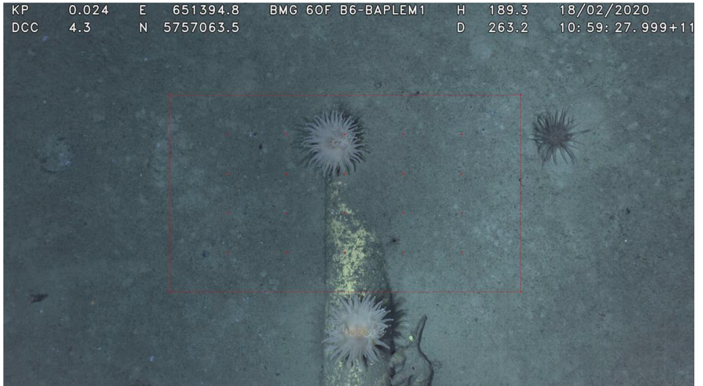
Figure 6-1 - Image from 2020 GVI showing the B6 Oil flowline transitioning from above to below the seabed (Ierodiaconou, et al., 2021)
