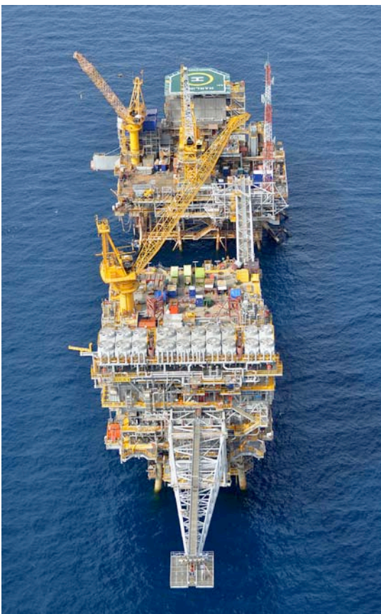
Figure 2 – Marlin B platform in foreground (existing Marlin A platform in the background)
