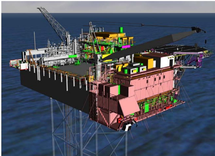
Figure 2-4 Yolla Platform with accommodation module
