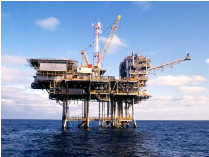
Figure 2 Barracouta platform (BTA)
