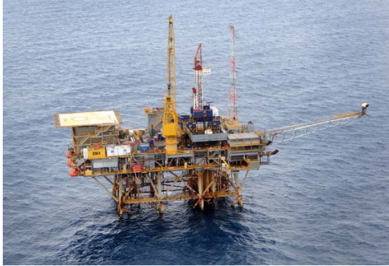
Figure 2 Bream A platform (BMA) (pictured with a drilling rig on board)
