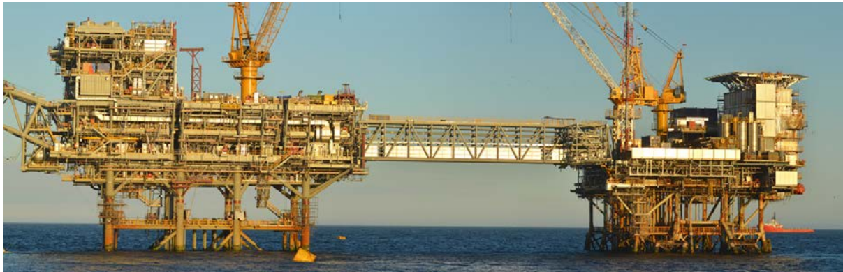
Figure 2 Marlin B Platform (left) connected to Marlin A Platform
