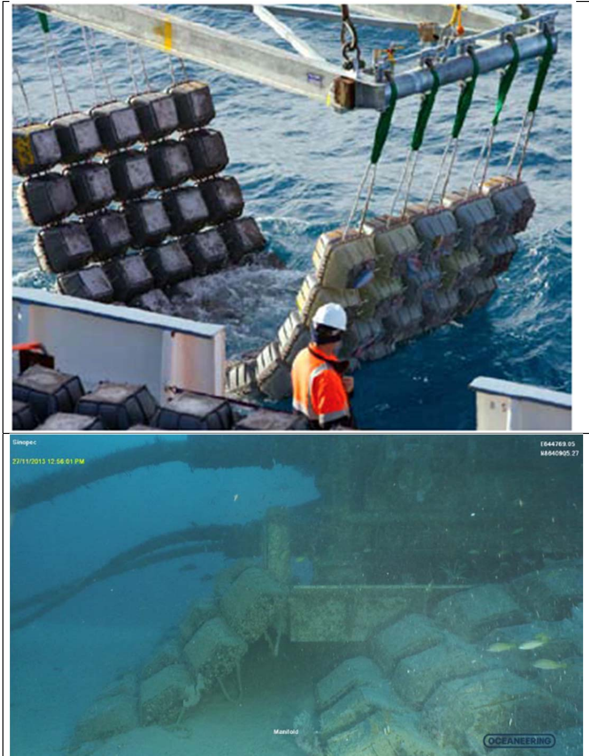
Photo 7. Concrete mattress; during installation (typical) and 2013 ROV survey (visible at base of manifold)
