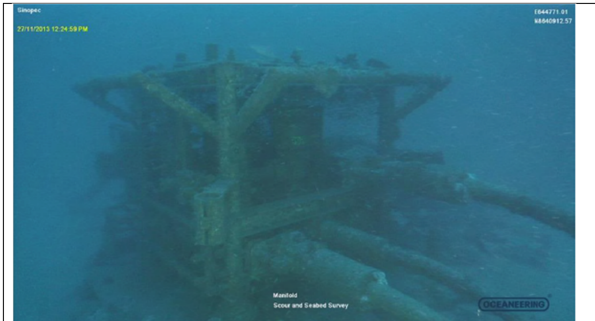
Photo 2. North face of the manifold (foundation structure not visible) from the 2013 ROV survey
