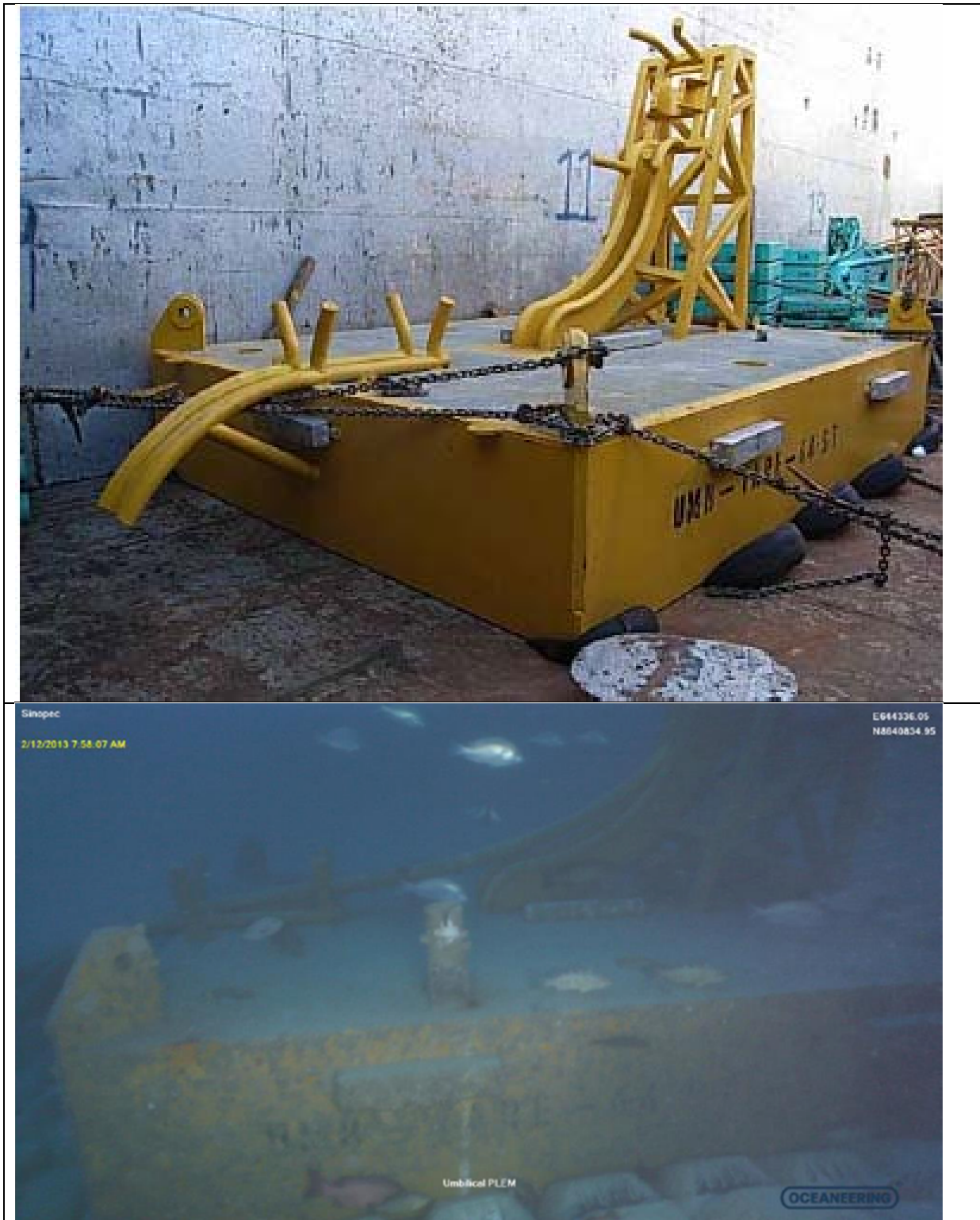
Photo 5. Umbilical PLEM; pre-installation and 2013 ROV survey
