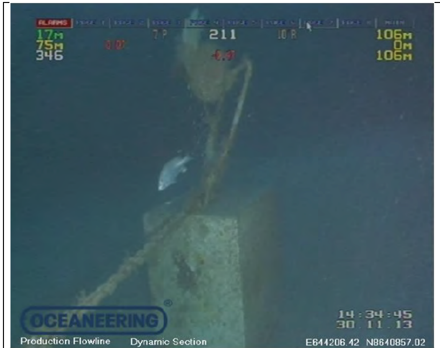
Photo 6. Typical riser clump weight (this one is connected to the production riser)
