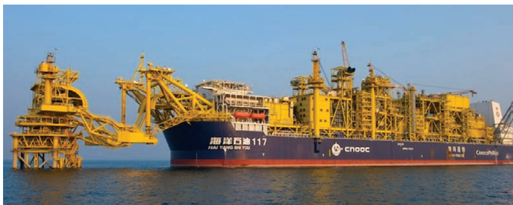
Figure 4-6: Example FPSO facility
