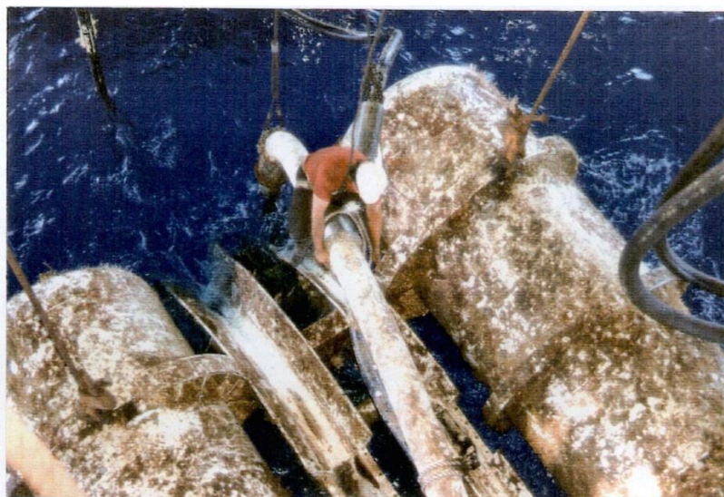
Figure 3-4 Decoupling of the T-7 flowline and umbilical from the buoyancy tank
