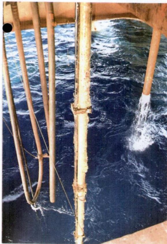
Figure 3-2 Recovery of T-1 flowline and umbilical through the rig moonpool
