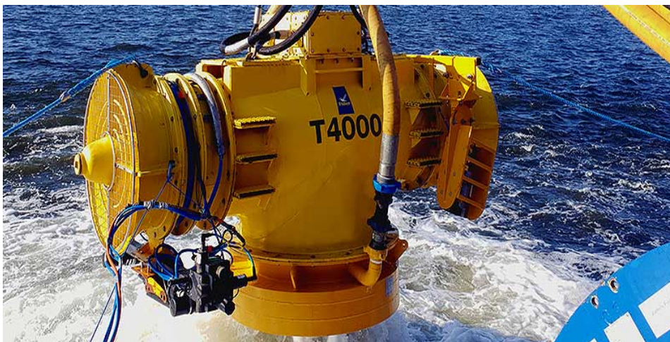
Figure 3-5: Example of equipment used for mass flow excavation
