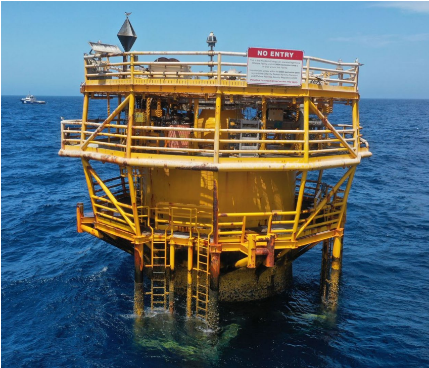
Figure 3-4: Topsides section of the RTM
