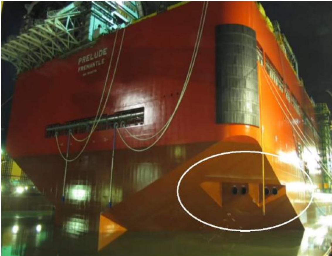
Figure 9-9: View of cooling water discharge ports P53, P54 (inboard pair), P63 and P64 (outboard pair) that discharge rearwards on the starboard side
