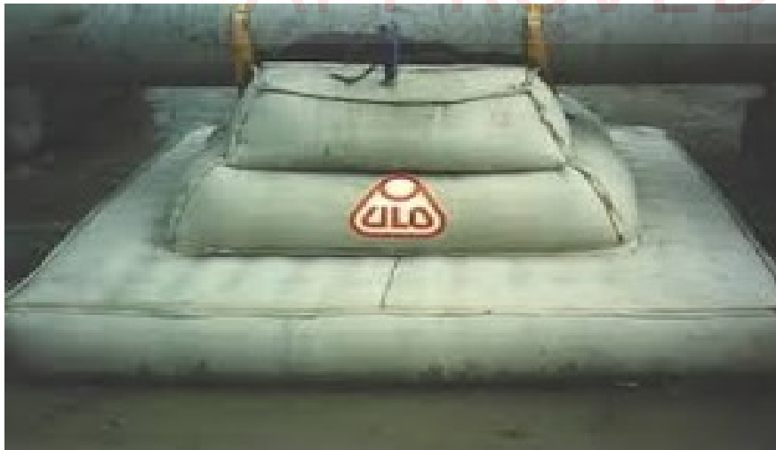
Figure 3-5: Example of grout bags
