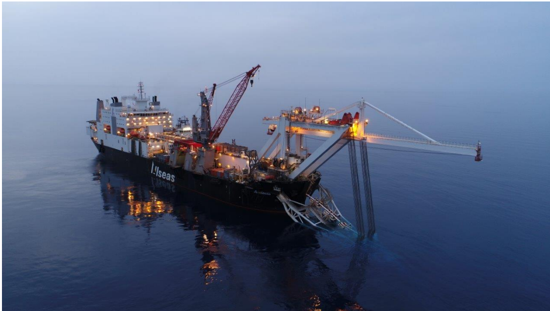
Figure 5-13: Photographs of a typical pipelay vessel at dusk
