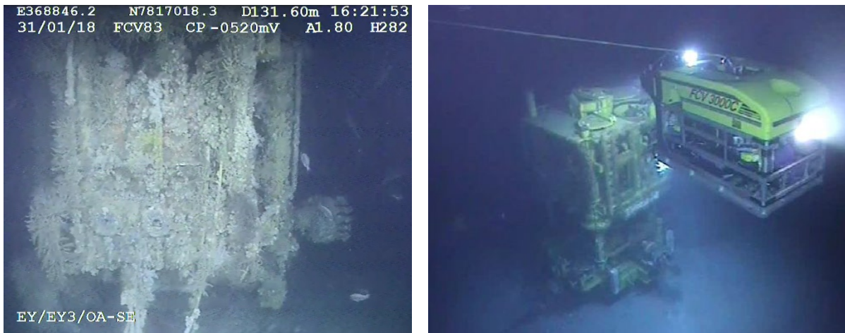
Figure 3-3: Left – Yodel-3 X-mas tree in 2018 ROV survey. Right – Yodel-4 X-mas tree in 2008 survey compared to ROV for size
