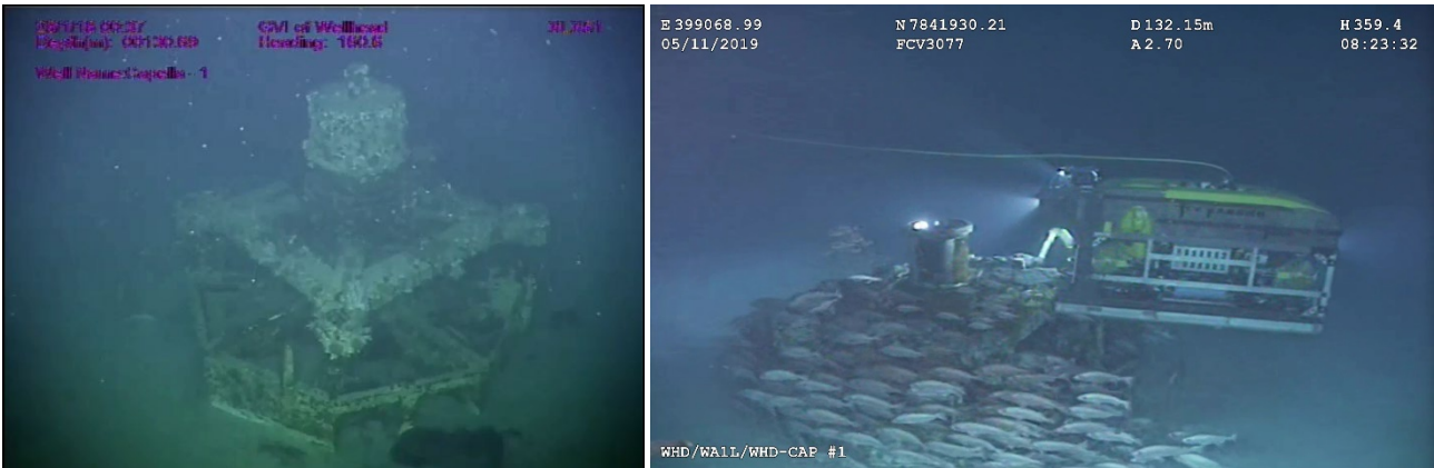
Figure 3-4: Capella-1 wellhead ROV images from 2018 survey (left) and 2019 (right)
