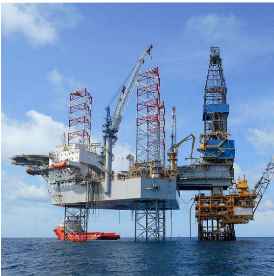
Noble Tom Prosser Jack-Up Drilling Rig (Image courtesy of Noble Corporation)
