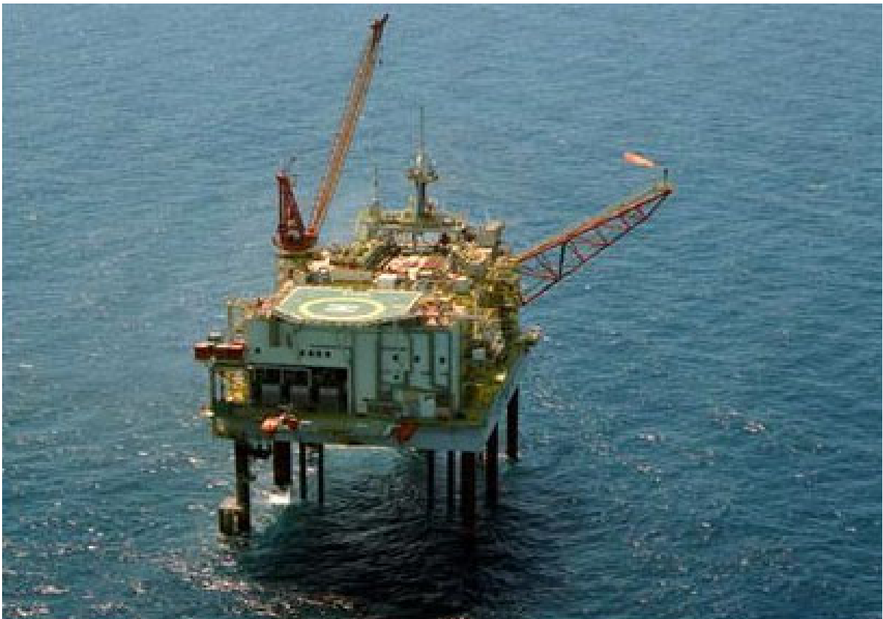
Figure 1-2: Aerial view of Stag Facility
