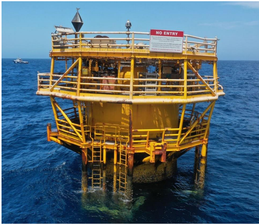
Figure 3-5: Topsides section of the RTM
