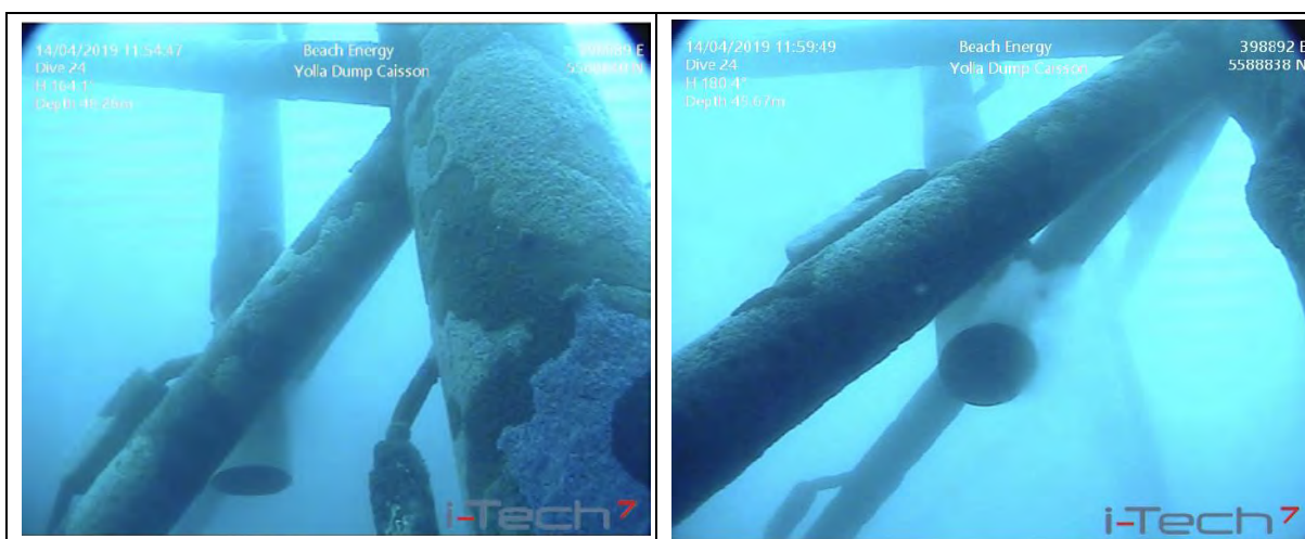
Plate 3.2. Views of the dump caisson from the 2019 subsea inspection campaign
