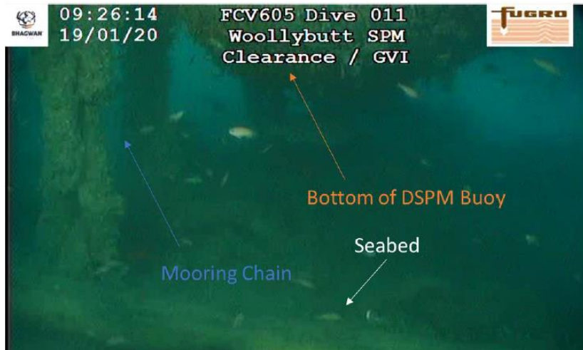
Figure 3-12: DSPM mooring chains
