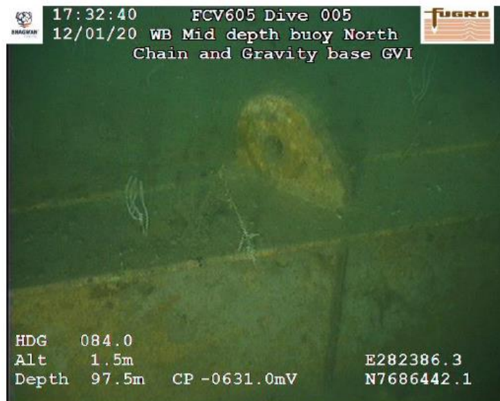
Figure 3-17: North MDB gravity base padeye
