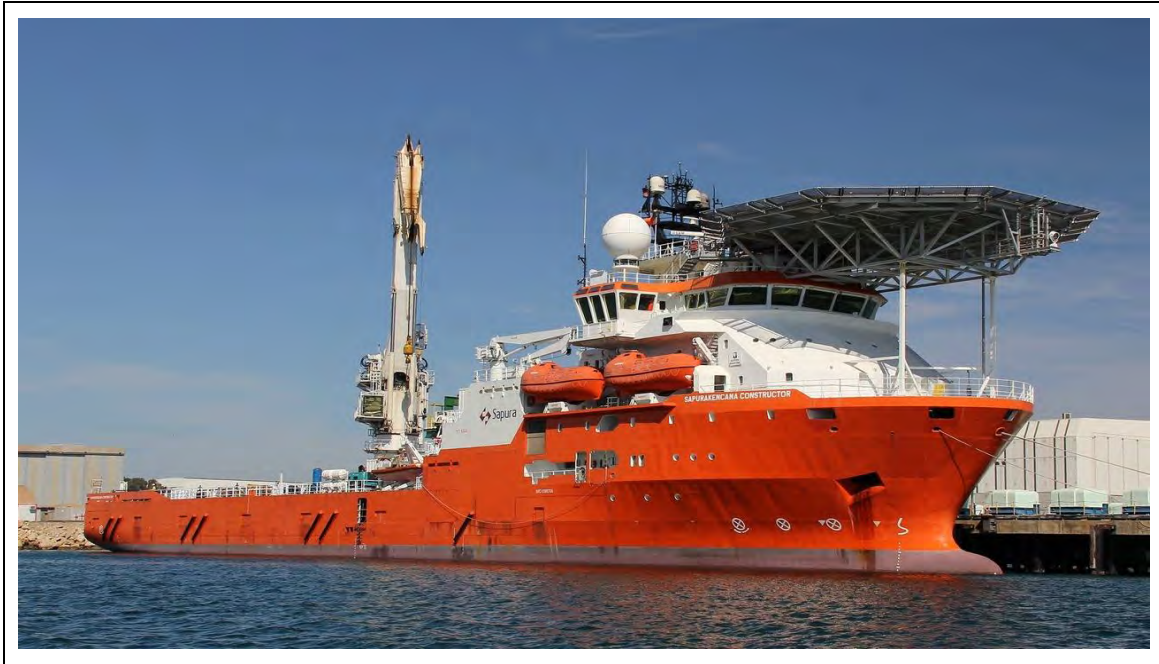
Photo 3.2. The MV Sapura Constructor offshore construction vessel
