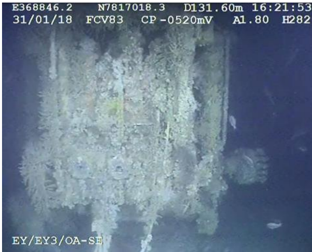
Figure 3-2: Yodel-3 X-mas tree in 2018 ROV survey
