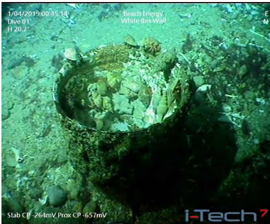
Photo 3.2. Close-up of the White Ibis-1 conductor
