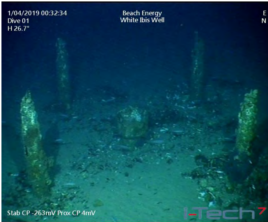
Photo 3.1. White Ibis-1 conductor and guide posts
