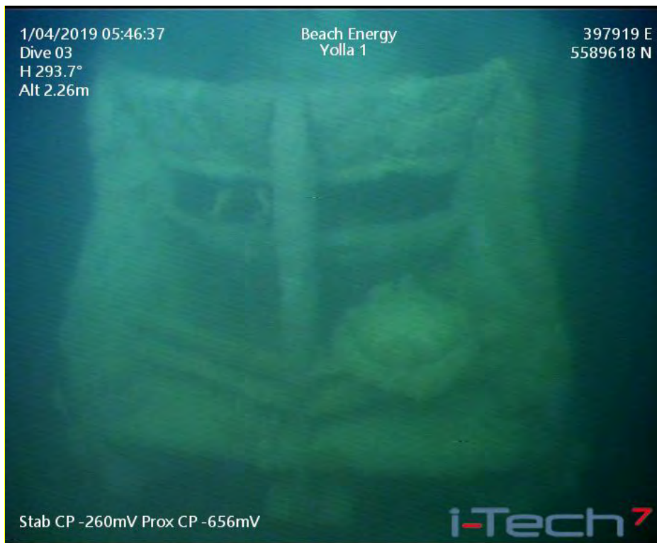
Photo 3.5. Yolla-1 wellhead overview
