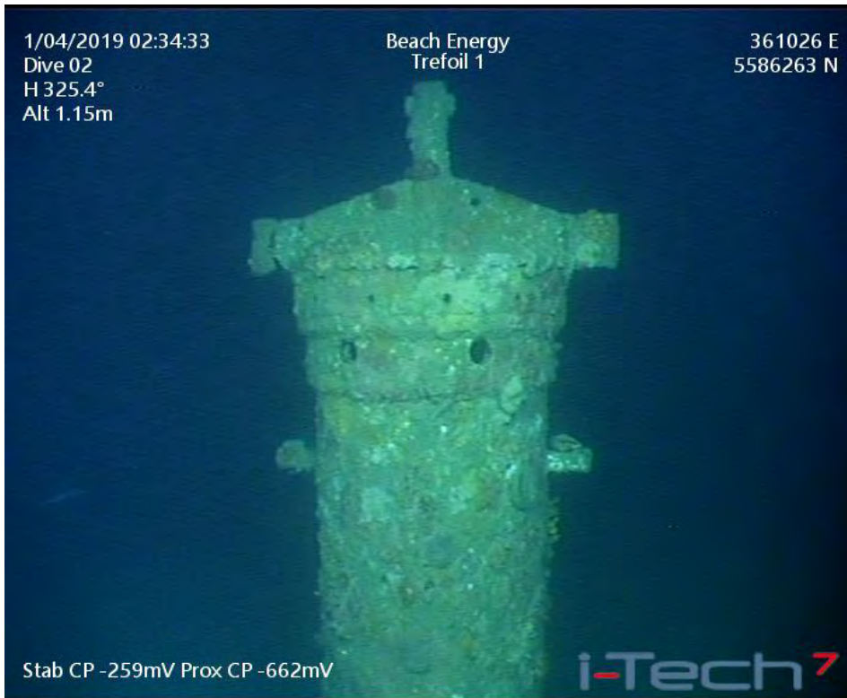
Photo 3.3. Trefoil-1 debris cap
